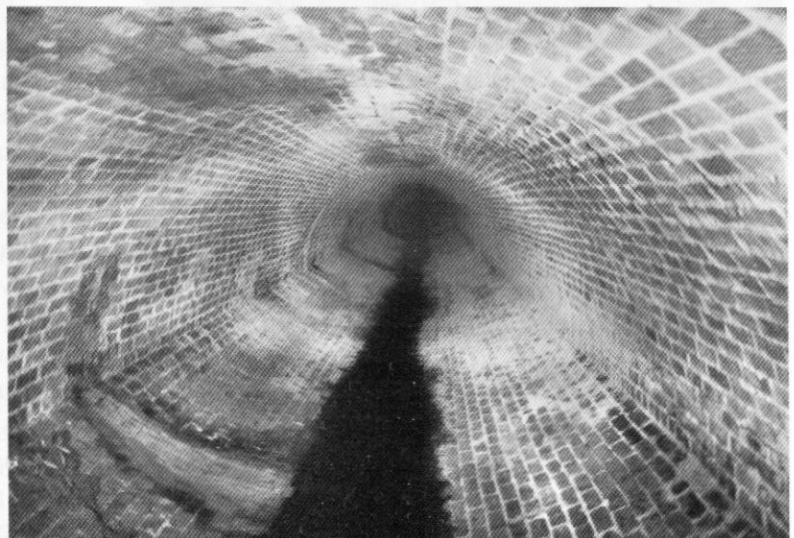
The overflow relief sewer. Photo Konstantin Binder
